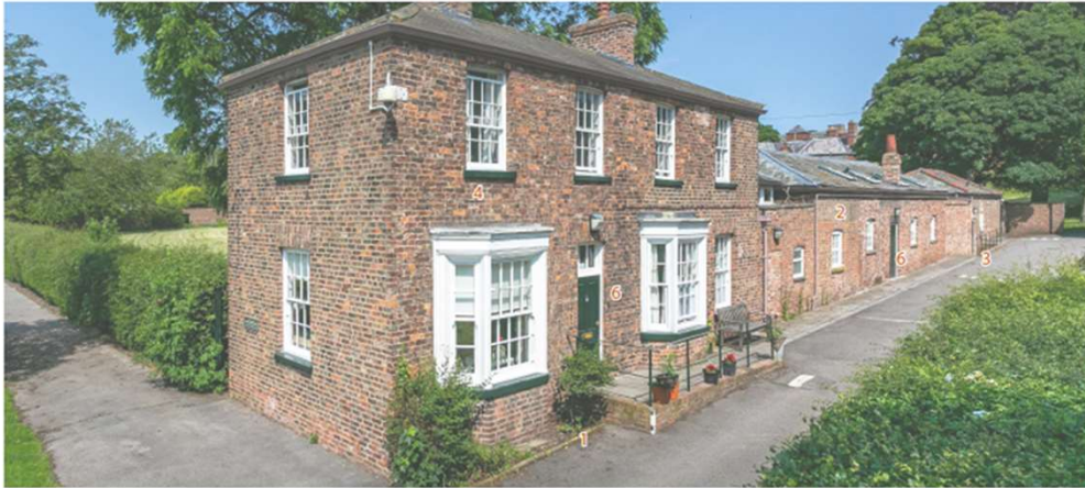
West Farm Range. South-West corner Jun 2020
